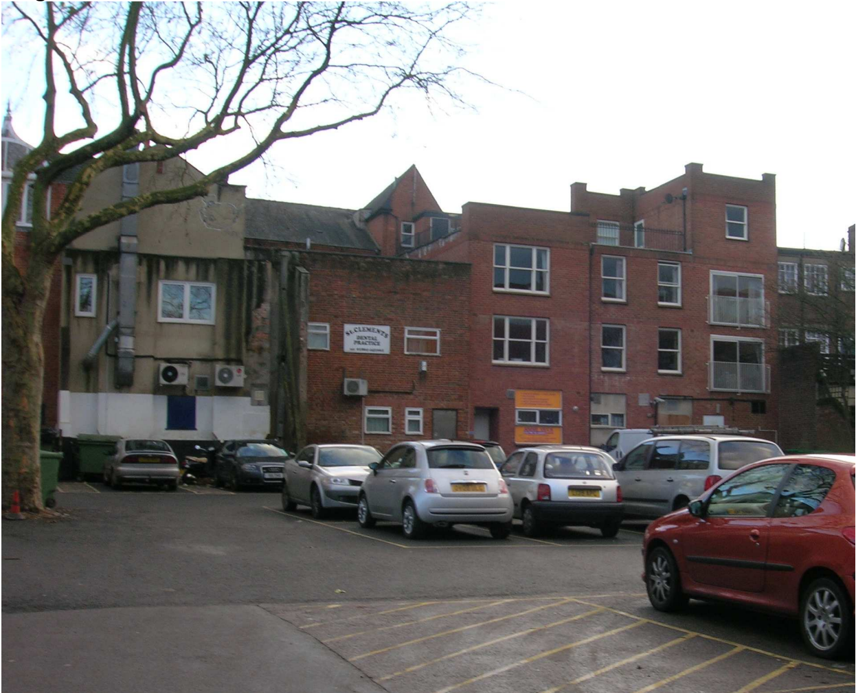
Figure 2: Rear of No 31-38 St Clements
